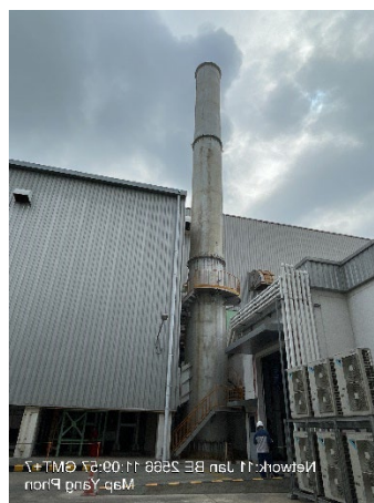
Fume Incinerator (2CPCL)
